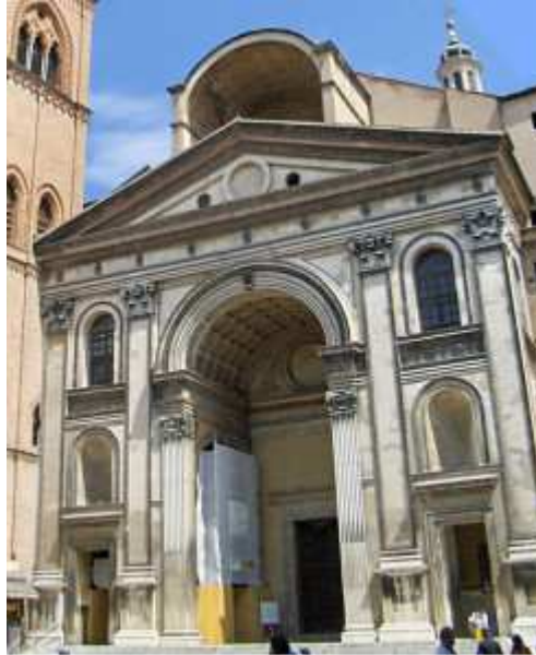
Fig. 12 Alberti's design for the facade of San Andrea (15th c.) in Mantua. Note the play on the classical triumphal arch theme (what amounts to three triumphal arches!) in the bottom zone and a classical temple pediment above. The barrel vaults, multi-story classical order pilasters, heavy cornices and niches are all characteristics of Italian Renaissance church architecture.
