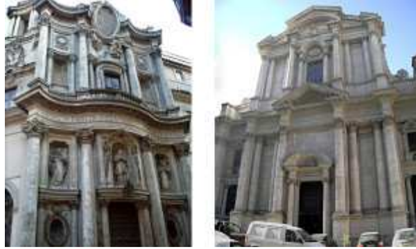
The facades of Baroque churches are treated like sculpture and appear more three dimensional than the flatter Renaissance style. Fig. 9 (L) Contrasting curved lines and forms often animate a facade. Niches with sculptures are common and cornices can be large, casting a dark shadow underneath. The curves and shadows create drama. Fig. 10 (R) Pediments are often broken by advancing and receding sections. Sometimes the center of a pediment is missing as is the one over the doorway, above. Once again the intention is drama and excitement.
